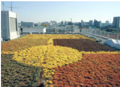
Example of an extensive green roof. Extensive green roofs require little maintenance and often feature grasses or other low maintenance plants.
