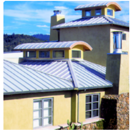
Metal roofs offer high reflectivity helping to mitigate the UHI effect. Source: Cool Metal Roofing Coalition
