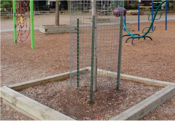
Wire mesh caging and t-bars prevent vandalism and damage to tree trunks.
