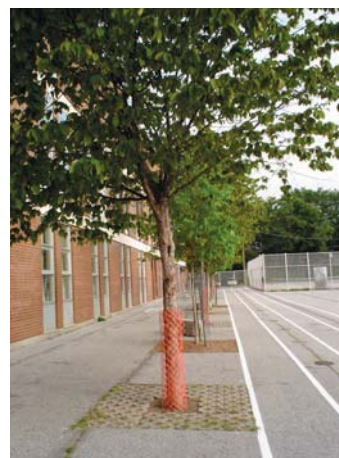
Trees planted in turf stone with snow fencing as protection. The permeable spaces allow water to seep through to the roots.
