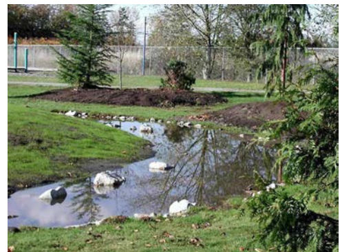
Bioswale for better drainage
